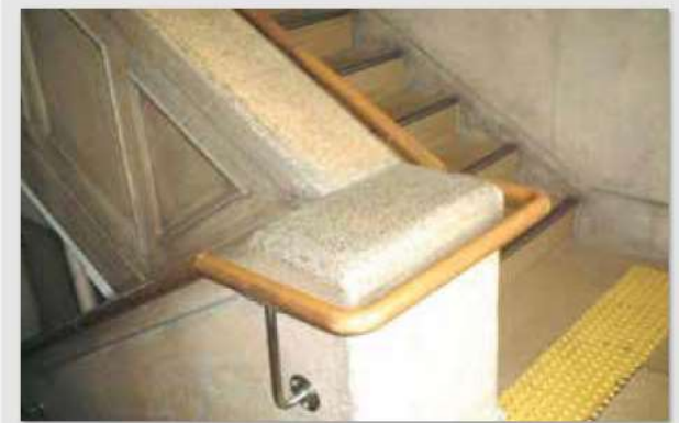
Handrail cover in municipal building (NPE)
