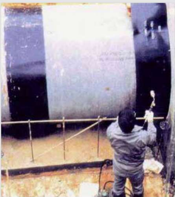
Waterproofing of Hume pipe joints with Nishi-Tube (NXL-A)
