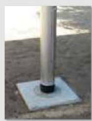
Example of corrosion prevention of lighting pole ground-contact points (NPM-A)
