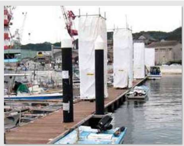
Corrosion prevention reinforcement for moored piles in Tamano City, Okayama (NXL-A)
