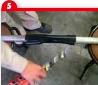
5 Use a burner, etc. to perform heat-shrinking. After shrinking, the rubber covering sheet may be peeled off.
