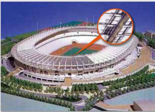
Overall view of Ajinomoto Stadium (NPE-Z)
