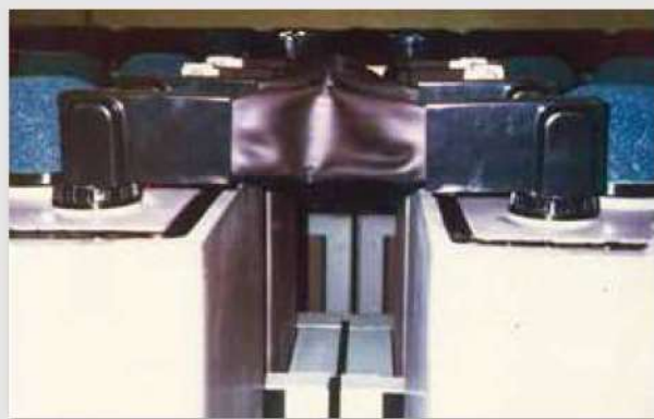
Flexible conductor insulating covering for batteries (NPE)
