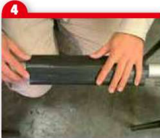
4 Apply a rubber sheet along the fastener part.
